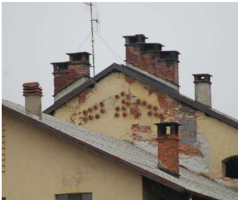
Figure 2: A cluster of bird pots on the wall of a dwelling (Biella, Italy)
