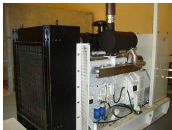
Fig. 1: One of three 100kW dutch generators at Garalo able to run on
