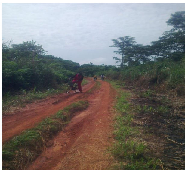
Plate 1.1 view of degraded road due to soil erosion
