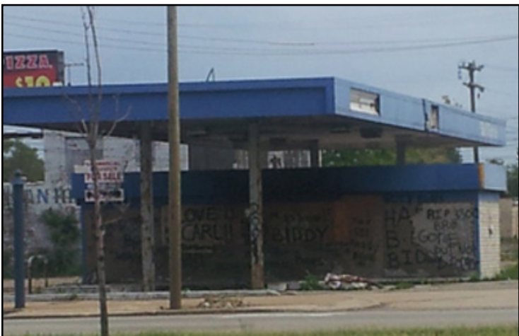
Vacant gas station on corner of Fort St and Schaefer to be demolished with this grant.
