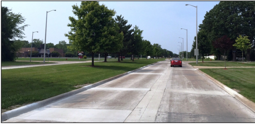
Complete renovation of Rancho Rd
