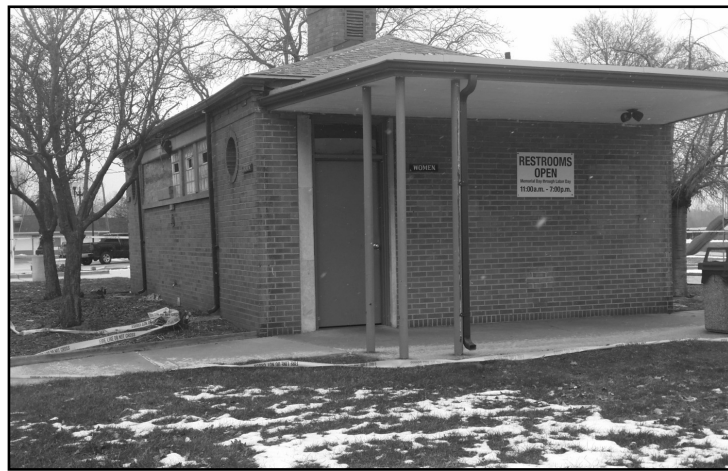
The bathroom facility at Dingell Park will be torn down
