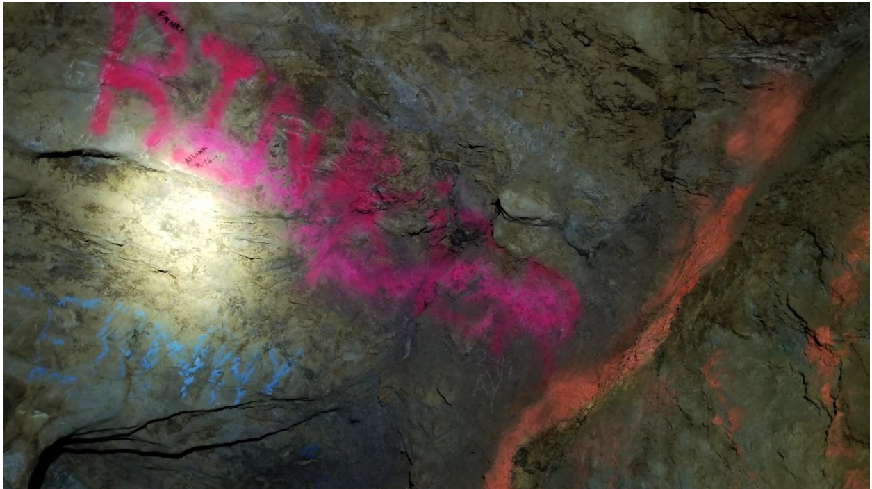
Book Room Area – Before restoration - Lusk
