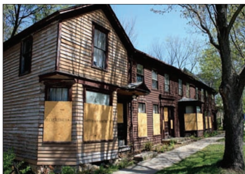
2012 Recipient: Israel Stowell Temperance House, Delavan, Wisconsin, to secure the structure before renovation
