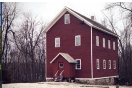
2012 Recipient: $500 was pledged to the Richfield Historical Society towards foundation restoration of the Messer/Mayer Mill.
