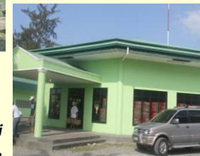
Construction of Multi Purpose Hall →
