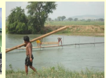
Construction of Footbridge at Barangay Kaingin & Vega ↓
