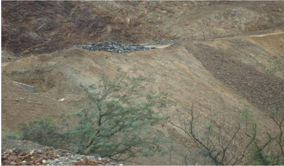
# 6, Quarrying and Road Construction in Brgy Labi
