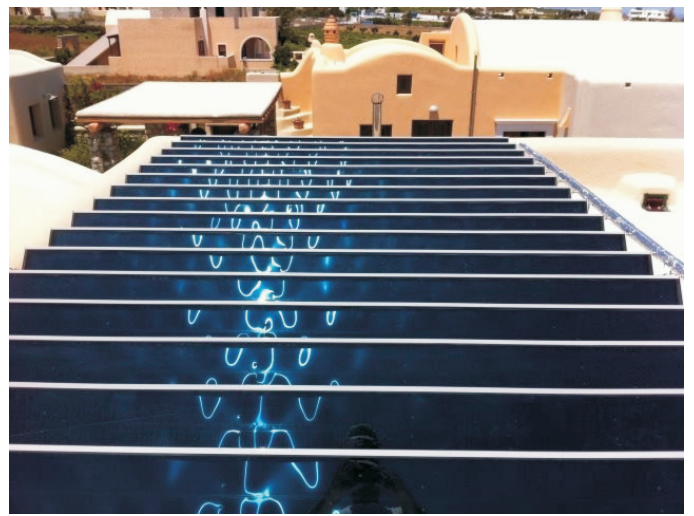
Panels can preferably be arranged in symmetric arrays. The hot water outlet pipe must higher than the inlet pipe.
