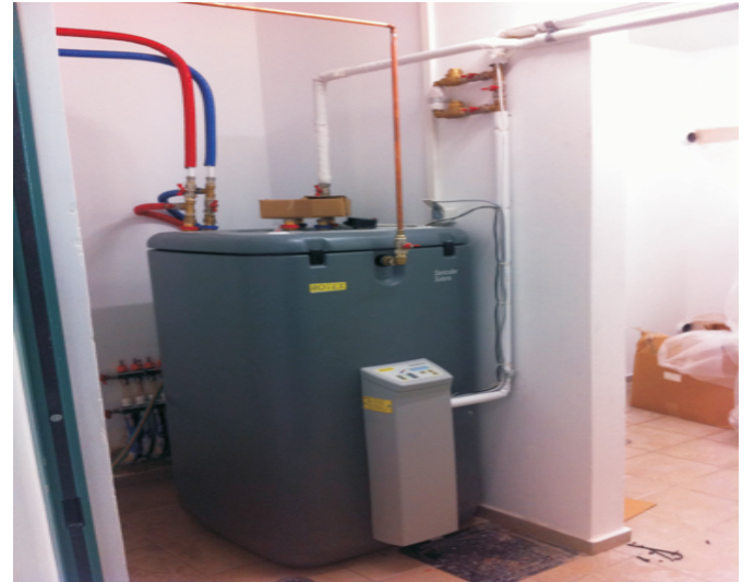
The non-pressurized solar water storage tank 500 L is well thermoinsulated to keep a mean temperature of 55-60°C.
