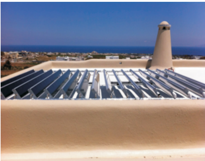
Panels are not affected by strong winds due to its free space the angle can easily be adjusted by turning in groups of four.
