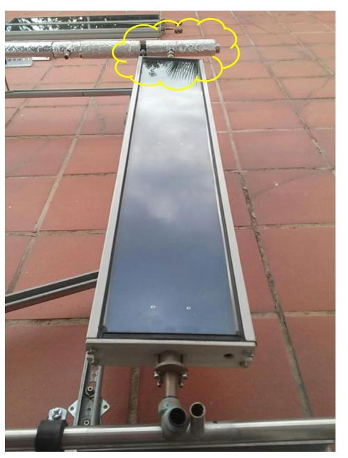
Mark the insert length on the SS-pipe to make sure that coupling is fully inserted
