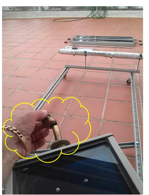
The 15 mm straight couplings are fitted onto the solar panels brass exit pipe
