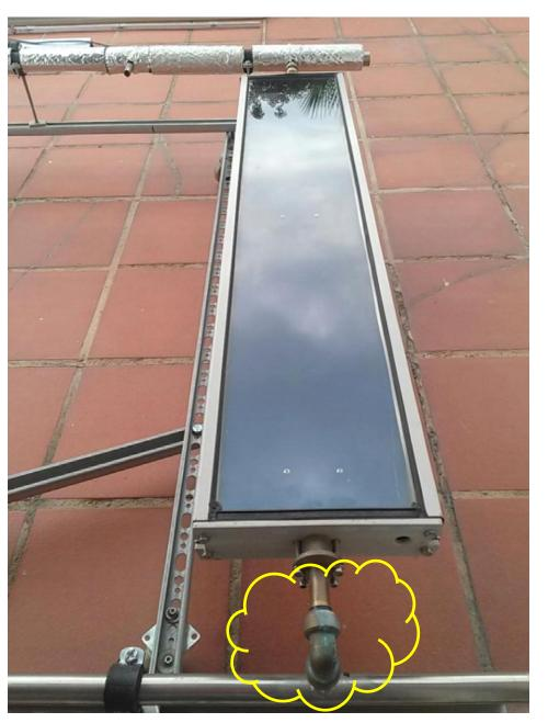
Mark the insert length on the SS-pipe and make sure that coupling is fully inserted
