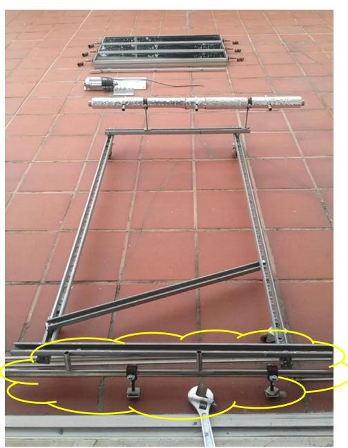
The water imlet manifold is always single sided with vertical outlet pipes 15 mm
