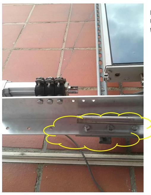
Pass the fixture and its square nuts in to the U-shaped fixing rail and tighten lightly the three 8 mm screws to hold in place
