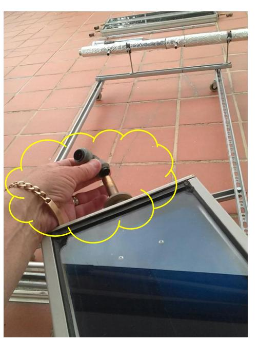
The 15 mm angled couplings are fitted onto the solar panels brass exit pipe
