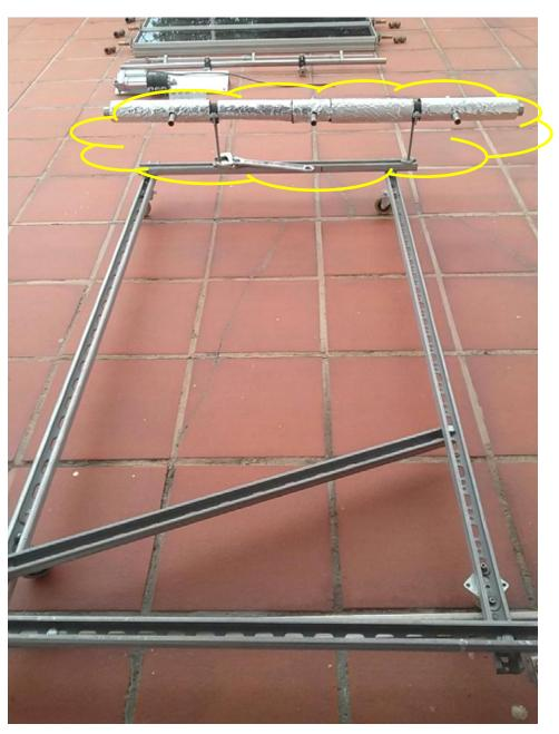
The water outlet manifold can be either single sides or twin sided (like on picture)
