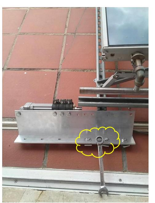
Bring the motor fixture into position
