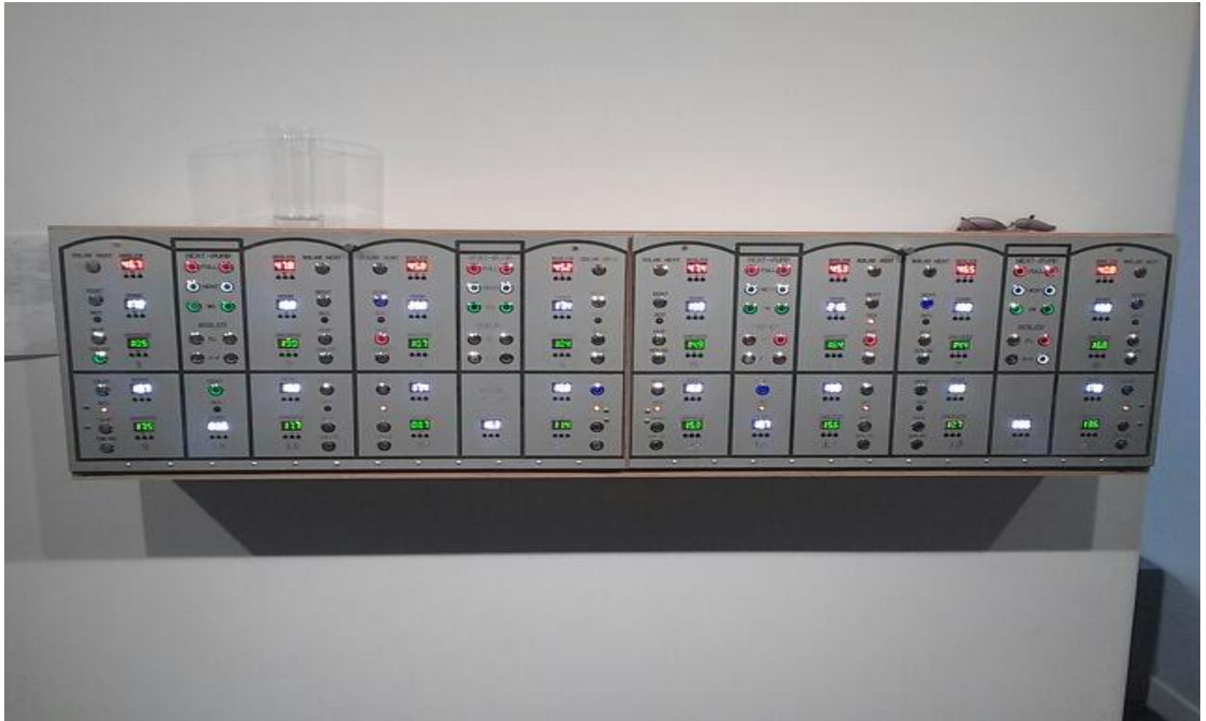
Control Board TP4-Enersol
