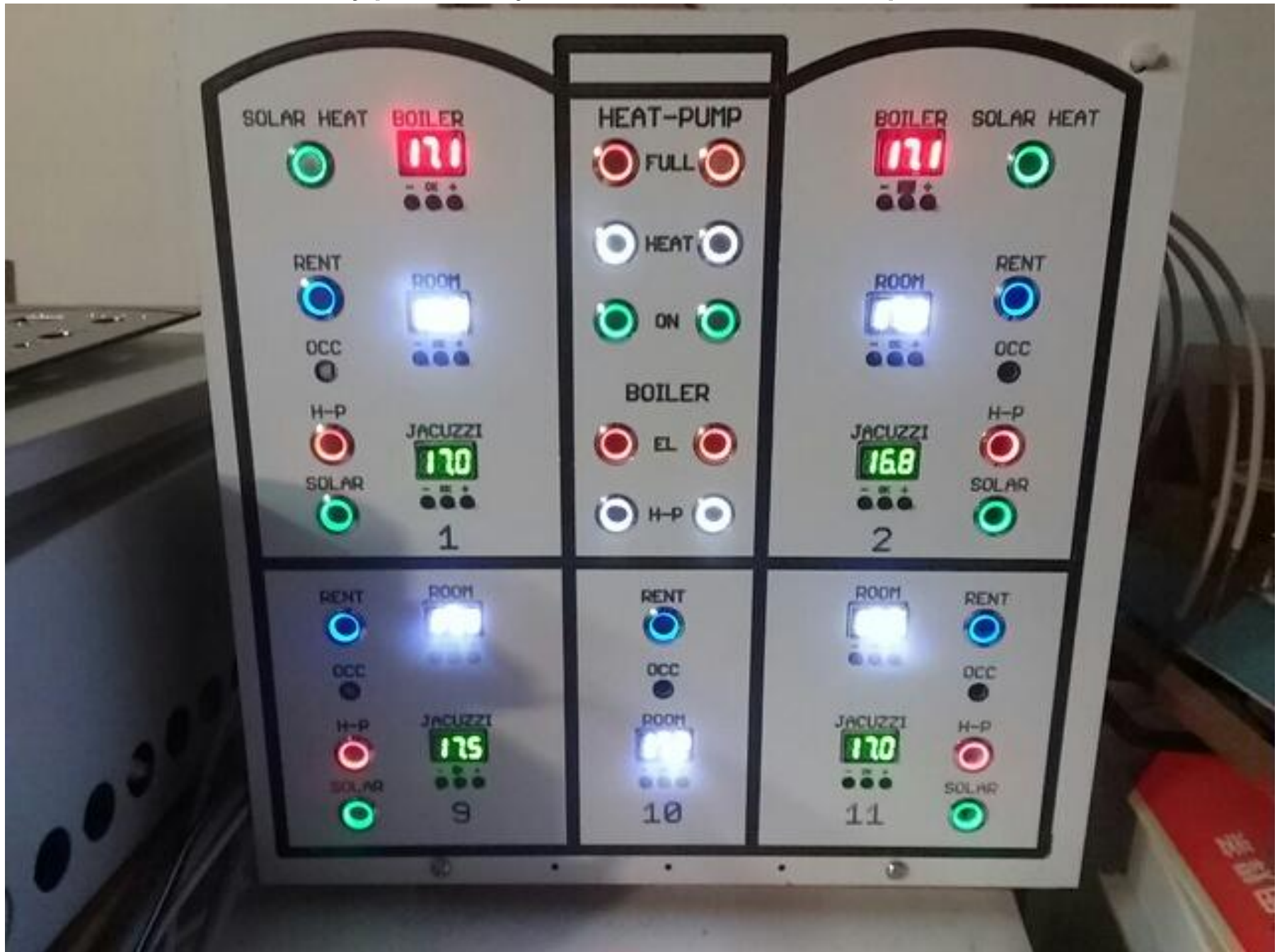
A typical layout of the control panel
