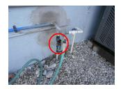
3. Acceptable Water Lines: CPVC, PEX Some or all water lines appear to have been re-piped with PEX and CPVC and copper stub outs, most of the plumbing in attic is not visible do to insulation.
