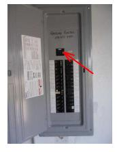
11. AcceptableBreakers: Copper12. Not PresentAFCI:13. AcceptableGFCI: At GFCI receptacles only14. Is the panel bonded? Yes
