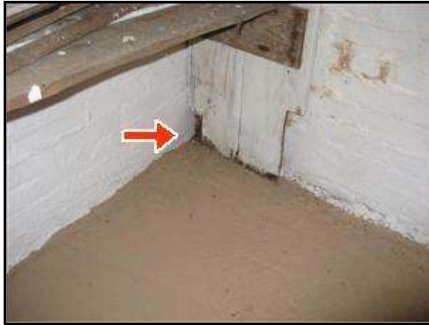
4.0 Picture 2 basement wall
