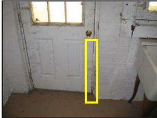
2.1 Picture 1 Basement entry
