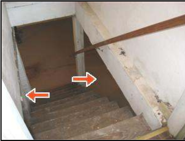
3.3 Picture 1 basement stairs
