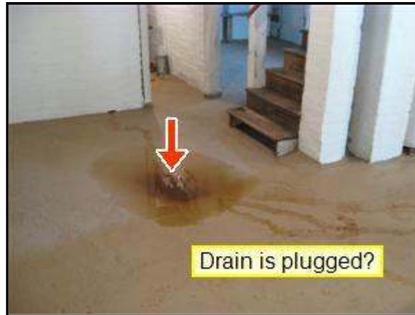
5.0 Picture 4 basement floor drain
