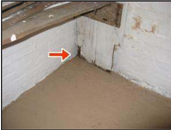
4.0 Picture 2 basement wall
