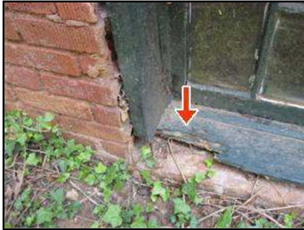
2.2 Picture 1 Basement window (s)
