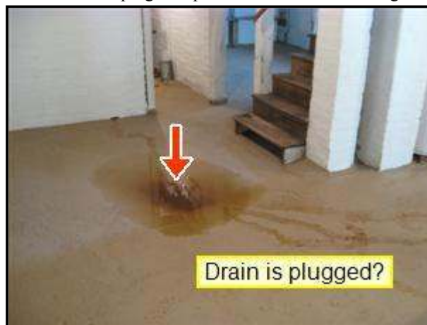
5.0 Picture 4 basement floor drain
