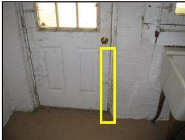
2.1 Picture 1 Basement entry
