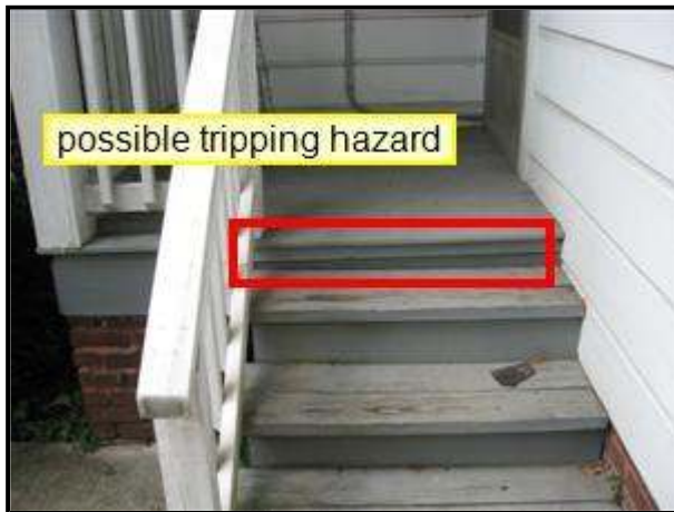
2.3 Picture 2 Rear Porch
