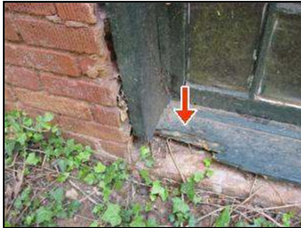
2.2 Picture 1 Basement window (s)
