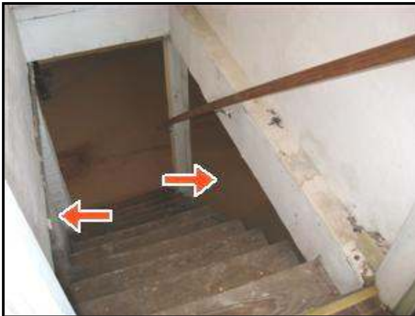
3.3 Picture 1 basement stairs
