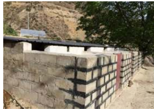
Cement reinforced pig pens made by trainees
