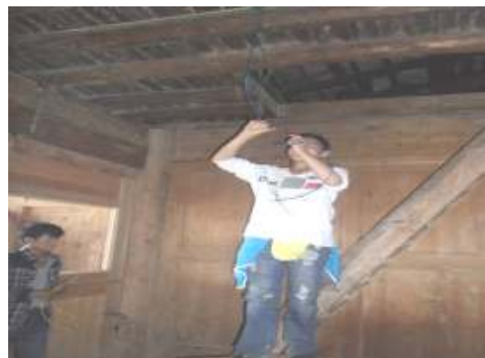
Trained electrician rewiring a house
