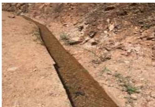
New cement lined canal for irrigation in Dong Wang
