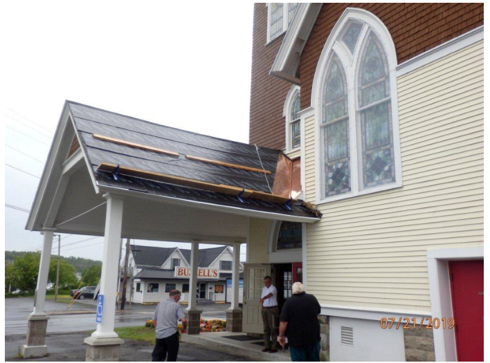
July 21 - roof replacement in progress on the portico!
