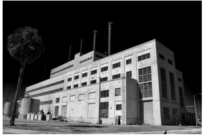
Florida Power Plant, Enterprise, FL
