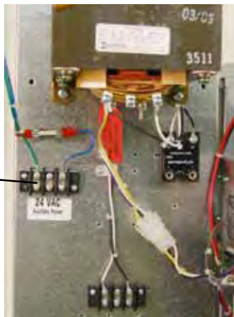
Figure 3-10 24VAC Transformer
