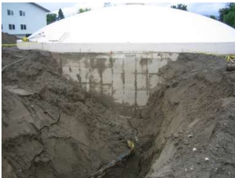
15 th Street 2B Reservoir: Exposed during 2005 Pipe Replacement
