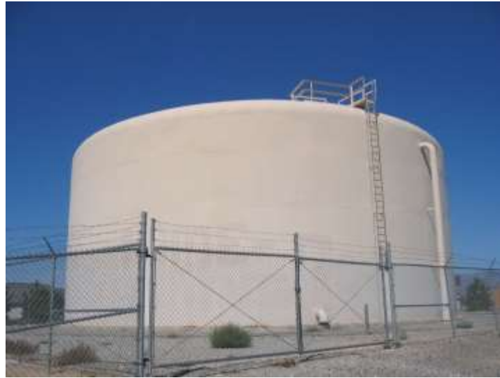
Fancher Heights Reservoir
