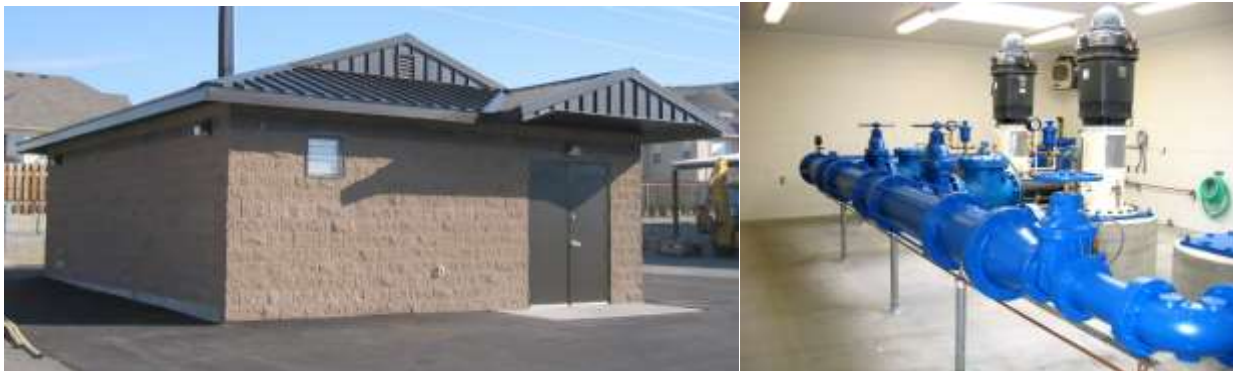
New 15 th Street Booster Pump Station
