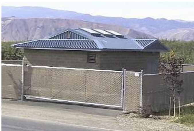
Grant and Nile Booster Pump Station
