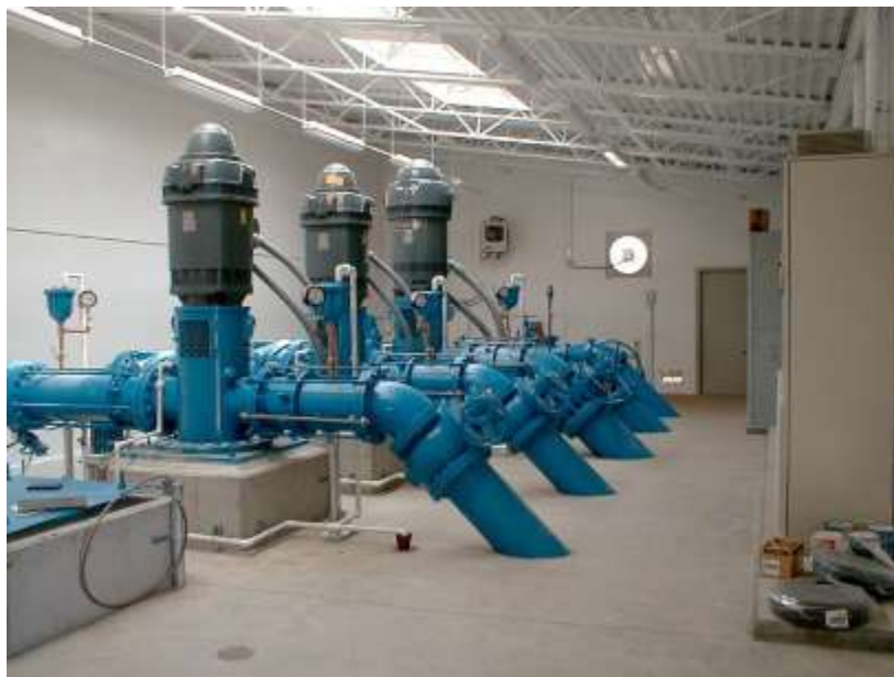
Regional Supply Station 965 Zone Pumps
