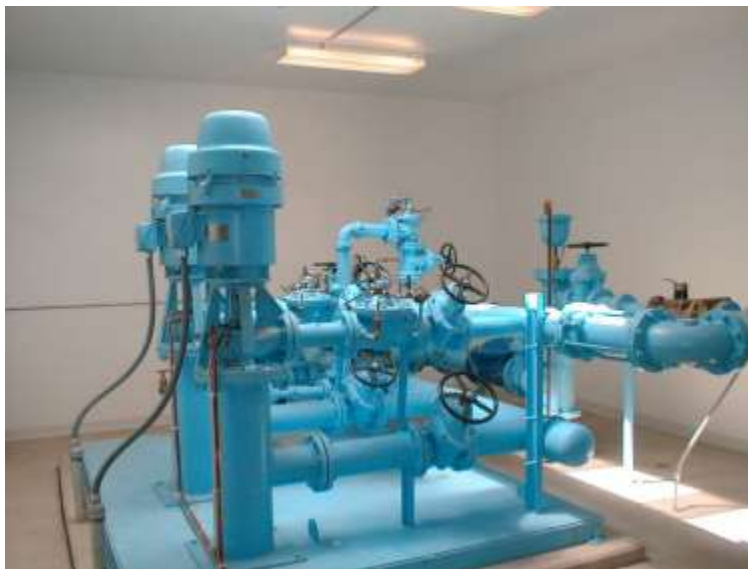
Canyon Hills Booster Pump Station
