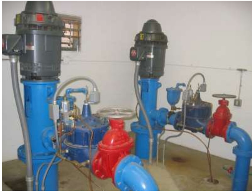
Daniels Drive Booster Pump Station
