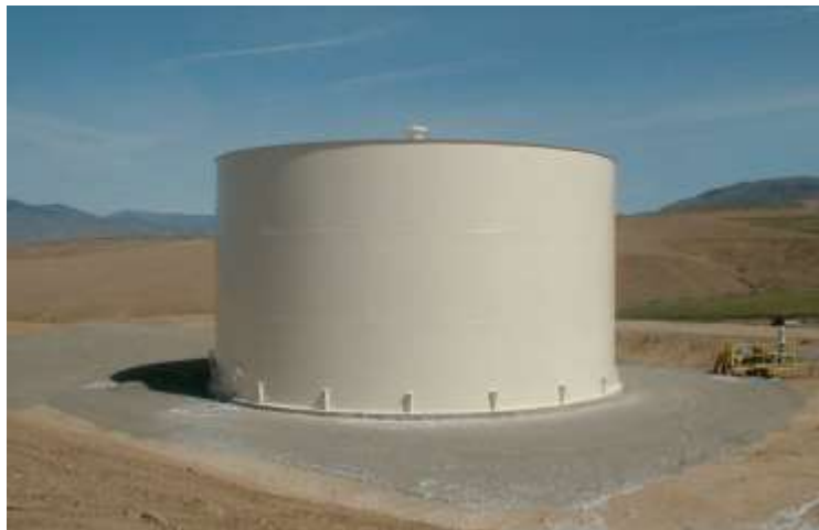
Canyon Hills Tank
