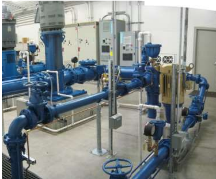
Regional Supply Station 1170 Zone Pumps
