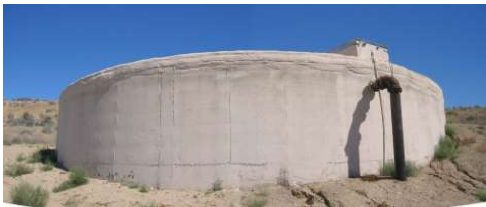
10 th Street 6A Reservoir
