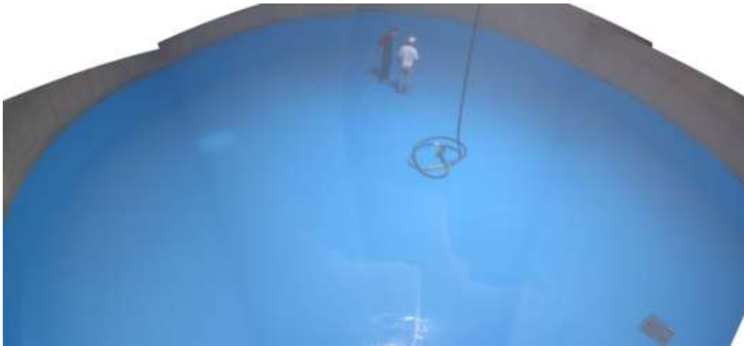
10 th Street Tank 6B Reservoir Internal Coating
