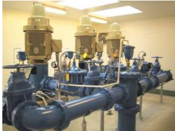
5 th and Grover Booster Pump Station
