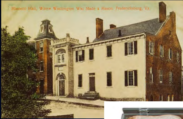
Fredericksburg Lodge #4 Hall
