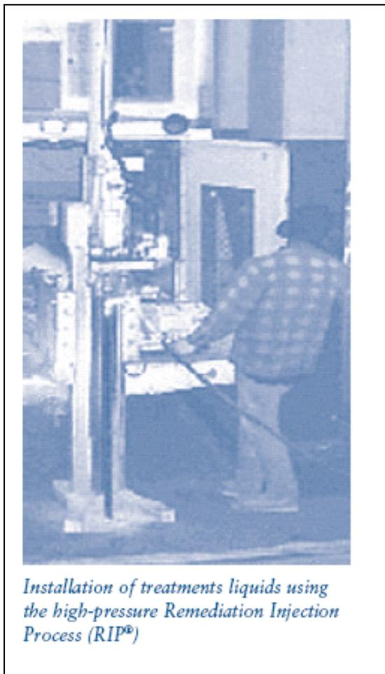
*Installation of treatments liquids using the high-pressure Remediation Injection Process (RIP®)*
